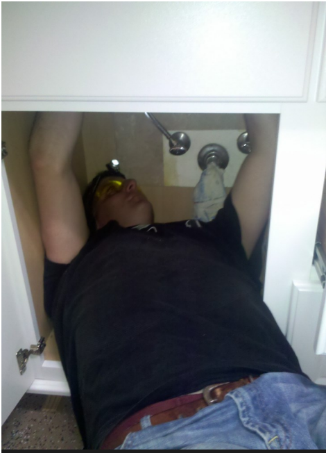
Pastor Steve Fixes Plumbing
